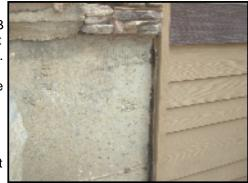
attain the recommended 6". It is important to maintain some clearance so that you can keep an eye out for signs of wood destroying insects.
