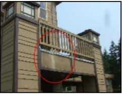
edge and onto the deck and stairway below. This entire deck surface and water proofing membrane below will likely need replaced to make it water tight as designed. Recommend a licensed contractor specializing in patio coverings and water tight membranes further evaluate and repair as needed.
