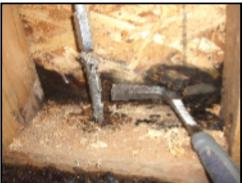
licensed drainage contractor further evaluate and repair the water penetration issues and a licensed contractor replace the damaged materials.
