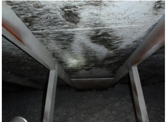
Fungus/Wood decayed roof sheathing.
